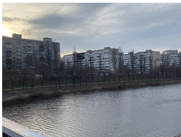
Image 1. View of the building hit by a Shahed drone during the night. Kyiv. November 2025
